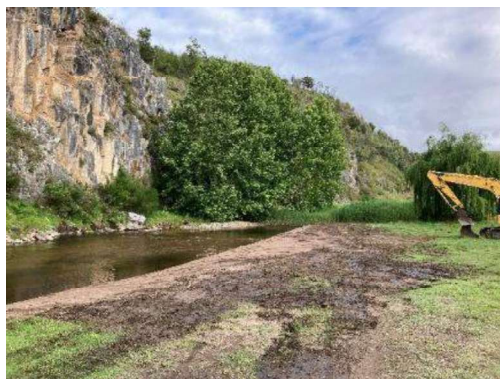
Completion of mechanical work at Buchan Bluff Reserve swimming hole
